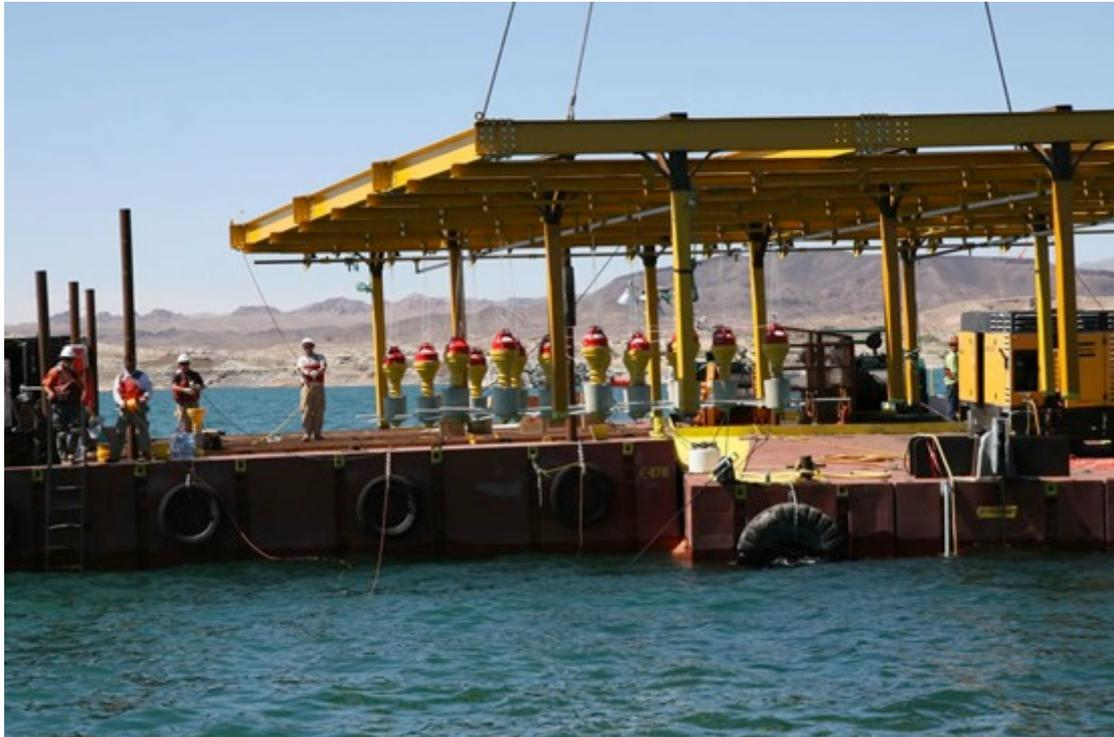
**Shows explosive frame ready to be lowered and accurately positioned using sonar on board the Falcon**
