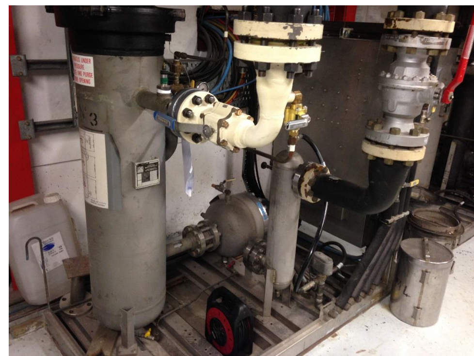
HCU-ER without temperature and humidity control
