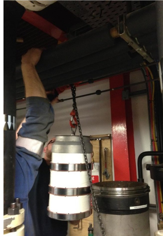
Hoisting ExtendAir® cartridge assembly into HCU
