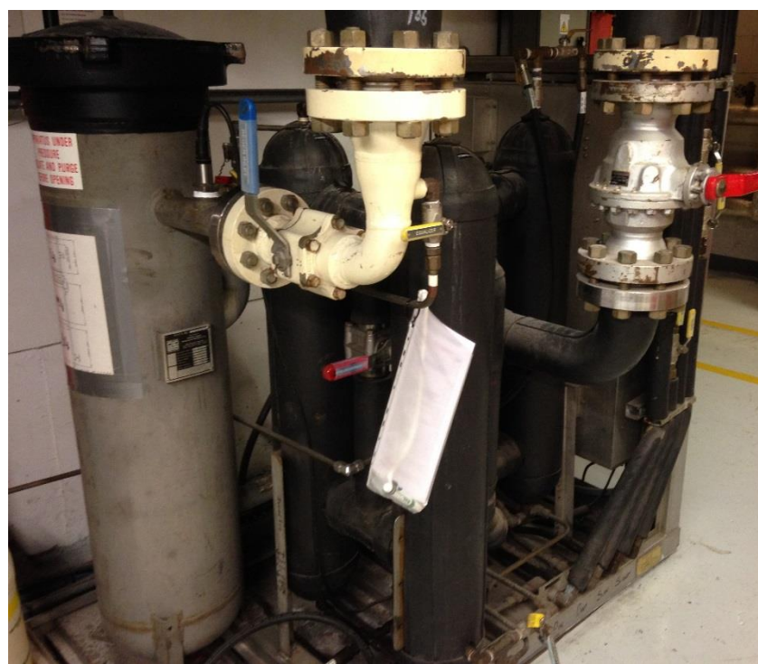
HCU-ER with temperature and humidity control
